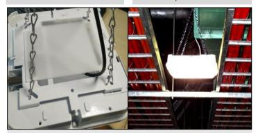
5. Alternatively the fitting can be suspended from the ceiling. A Smart-Connect Base plate with a 3m flex & plug suitable for hanging is available for purchase separately from enLighten Australia. Attach the chain to the base plate (as shown above) and plug the 3pin plug into a power socket or hardwire it into a junction box.
