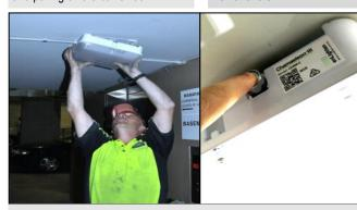
4. Place Smart-Connect Base plate hinge tabs into slots located at opposite end to barrel lock. Align the electrical connector terminal pins on the light fitting to the terminal block sockets on the base.
