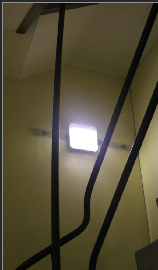
Fire stair - Chamaeleon light in standby mode
