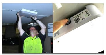
4. Place Smart-Connect Base plate hinge tabs into slots located at opposite end to barrel lock.
