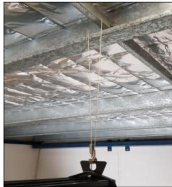
3. Loop the stainless steel cable around the beam and clip the other hook into the bracket
