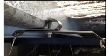
3b. Mount single point mounting bracket onto a purlin clip (not included) and secure onto purlin
