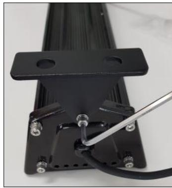
Connect the surface mount brackets onto each end using a 4mm Allen key (30W—150W models). Then mount the fitting to the ceiling
