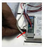
8. Plug battery plug into driver and note date of commissioning on battery.
