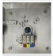
5. Connect building wiring to mains terminal.
