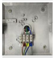
7. Connect Switched Active into SW terminal, Permanent Active into A terminal.
