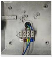
7. Connect wire loom from gear tray into the terminal block.
