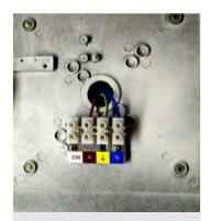
5. Connect building wiring to mains terminal.
